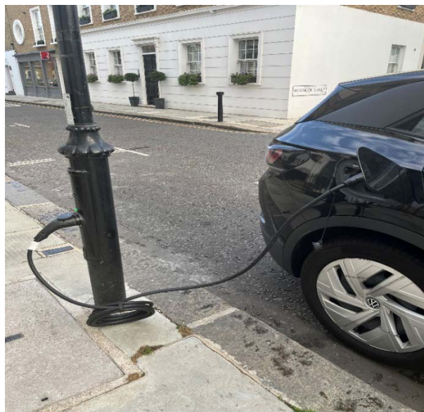
Figure 13. Mode 3 charging station built into a streetlight post with an untethered cable.
