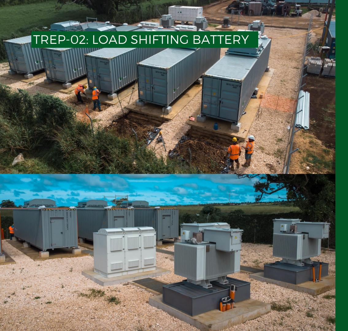
TREP 02 Load Shifting BESS civil and mechanical installation works complete
