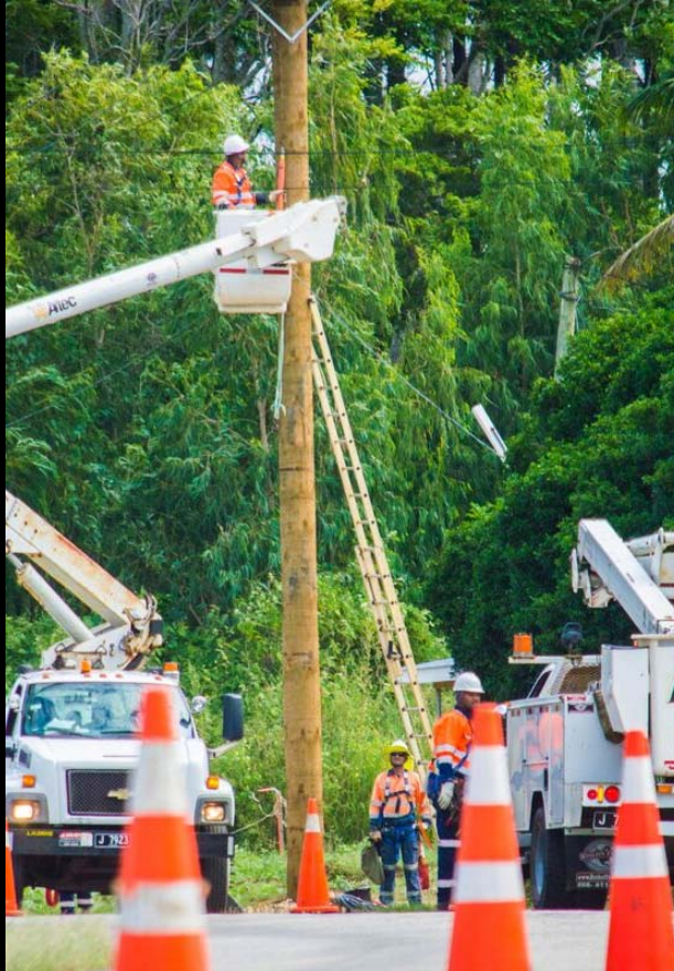
New Connections with homes and businesses not previously connected to the grid.
