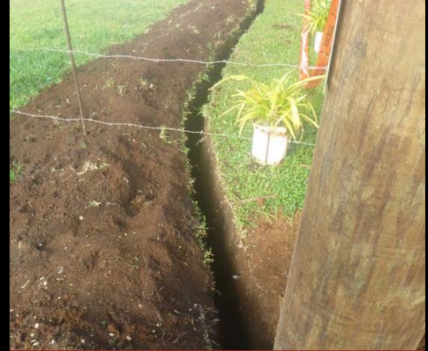
New underground service line to all premises providing free new connection
