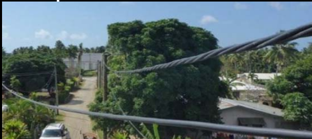
Upgrade Low and High Voltage within urban areas of Tongatapu
