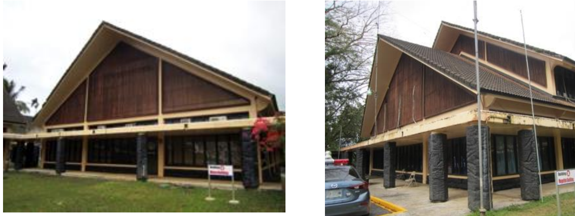
Figure 1-2: General View of the Facilities
